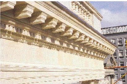
*Sandstone detail after repair with specialist mortar*
