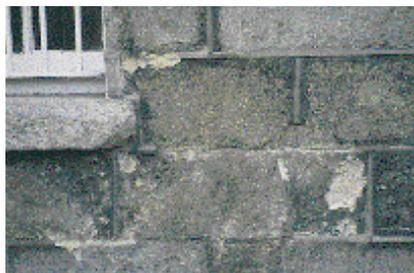
*Damaged granite, caused by inappropriate pointing.*
