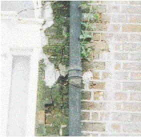
*Damaged brick work, caused by leaking pipe and over-dense pointing.*
